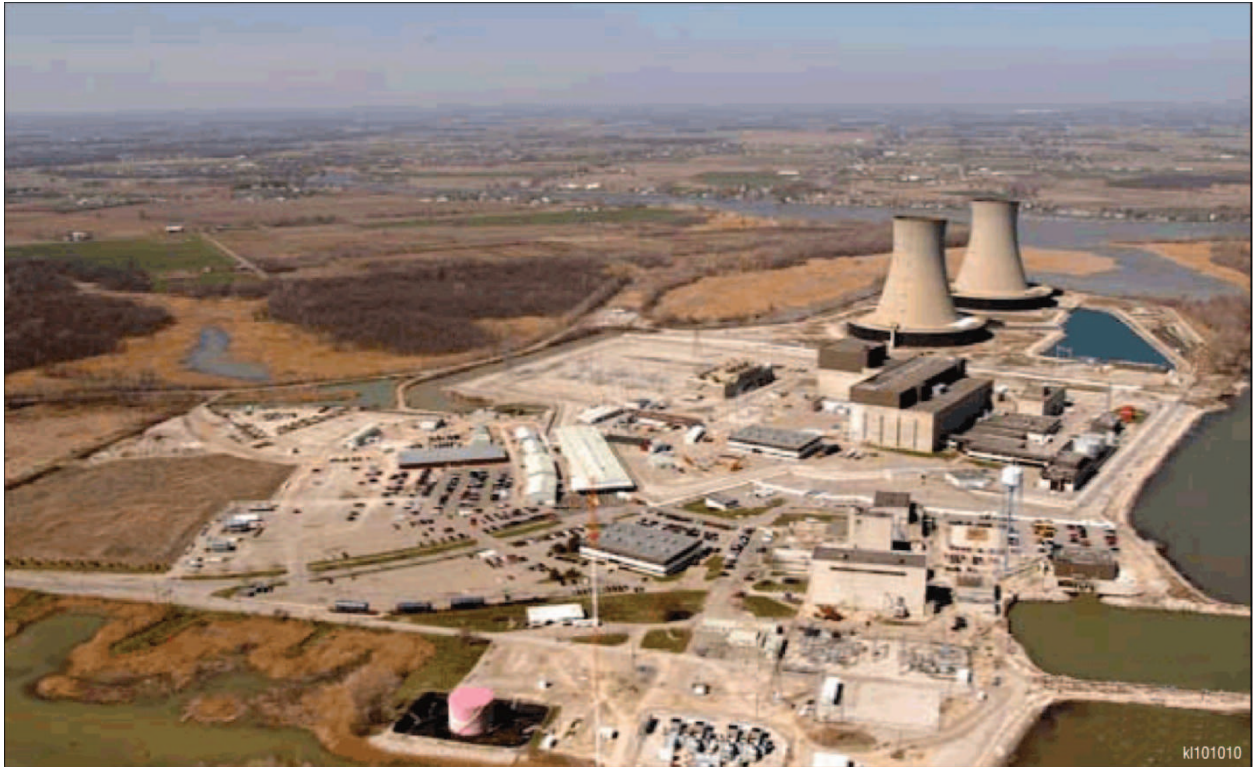
Figure 3-3. Aerial View of the Existing Fermi Site Looking North (Detroit Edison 2011b)
