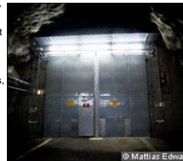
The waste facility at Forsmark power station, Östhammar
