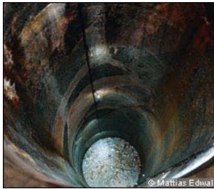
Canisters containing waste will be placed in clay-lined holes 450m underground
